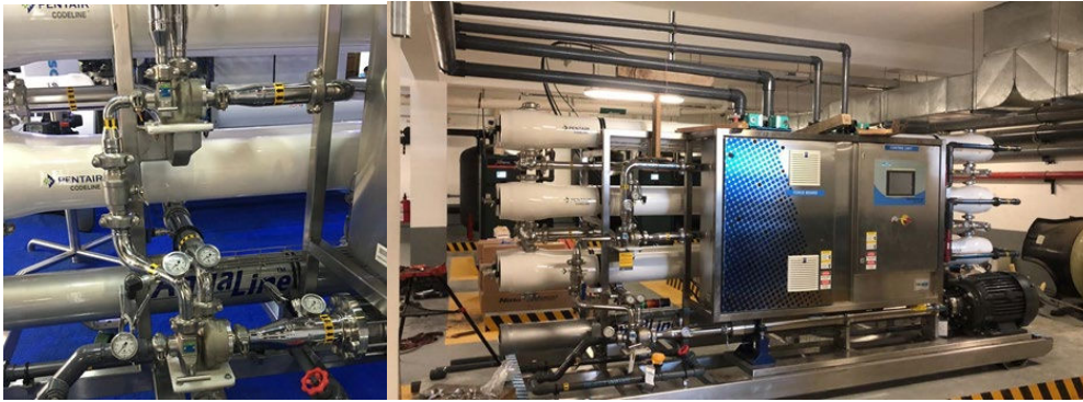
Figure 8: Biturbo™ skid and turbocharger arrangement (left) Feed turbocharger at bottom; interstage turbocharger at top (right) Full skid installed at Rancho San Lucas, Baja California, Mexico
